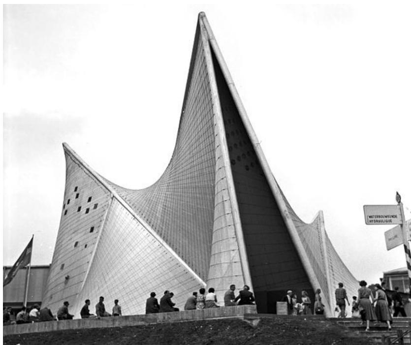
**Figure 3.18:** Philips Pavilion at the world expo 1958 in Brussels formed from hyperbolic paraboloids, designed by Le Corbusier and Iannis Xenakis for the performance of spatialized electronic music. [© wikimedia commons / Wouter Hagens]
