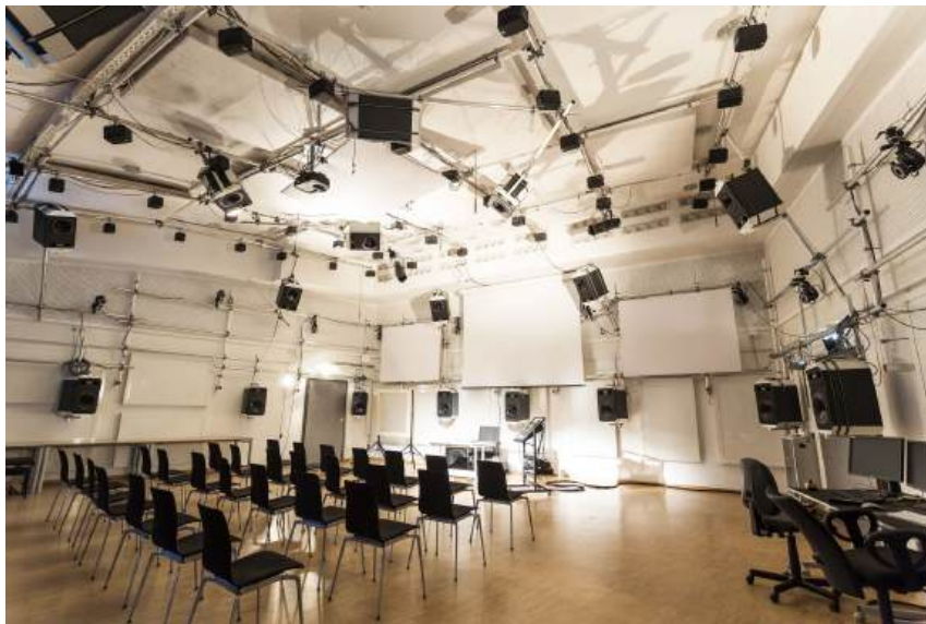
Figure 2: Example of a medium-scale spatial audio system: IEM CUBE with 24 point-source loudspeakers, Tannoy Systems 1200, mounted in a hemispherical arrangement, Photo: Wolfgang Hummer.
